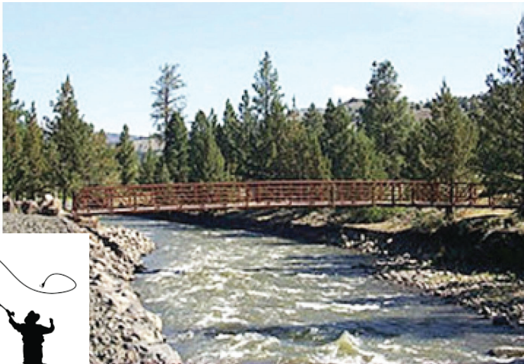
Foot Bridge across the Chewaucan River
