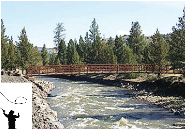
Foot Bridge across the Chewaucan River
