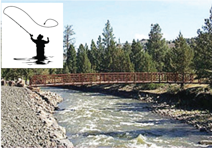
Foot Bridge across the Chewaucan River
